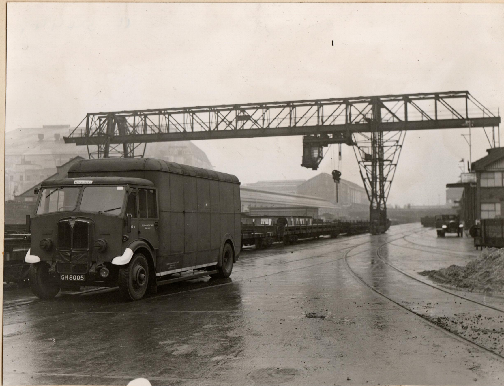
442 W - PER WAY (RLYS) BREAK-DOWN LORRY - LILLIE BRIDGE DEPOT
