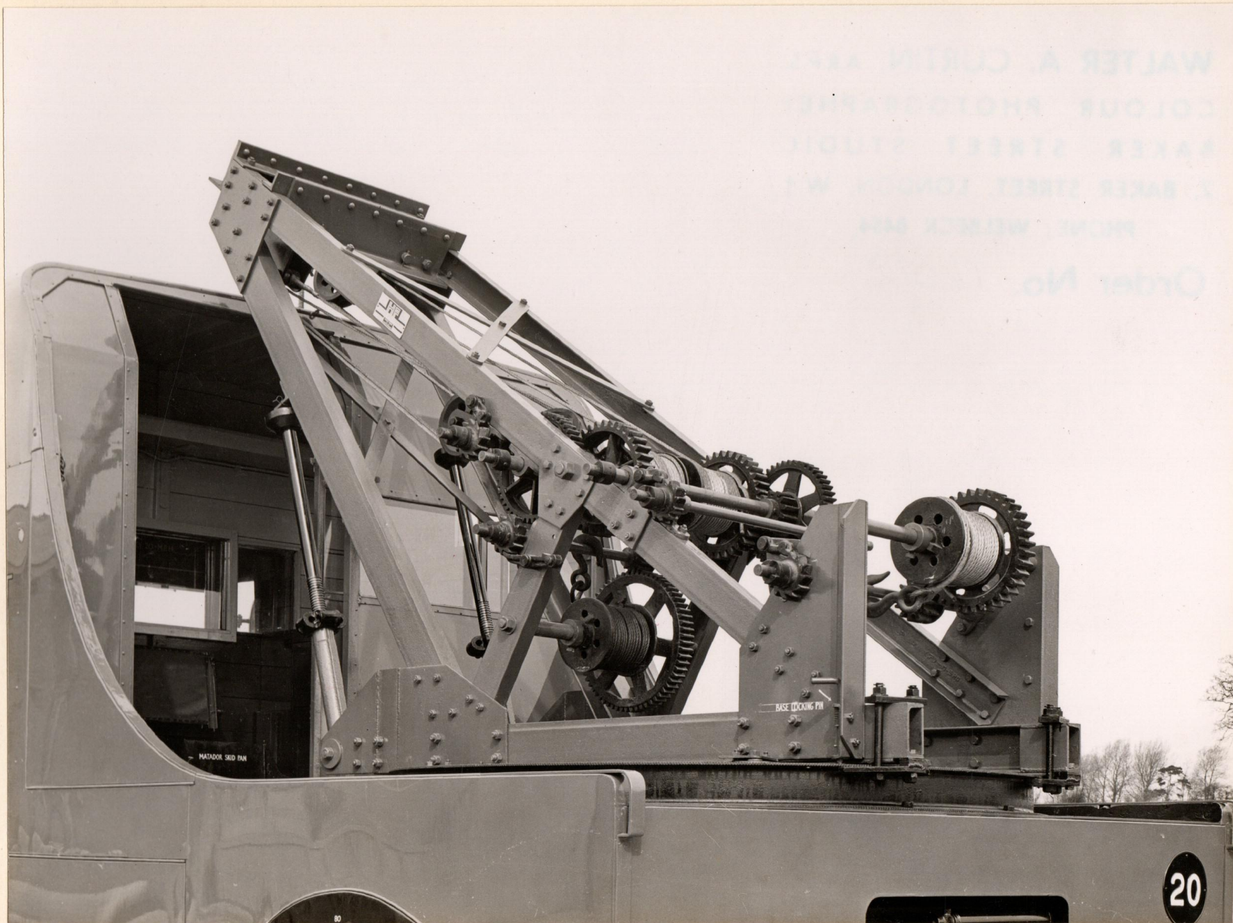
A.E.C. MATADOR BREAKDOWN LORRY WITH 5TON CRANE. 751P.
