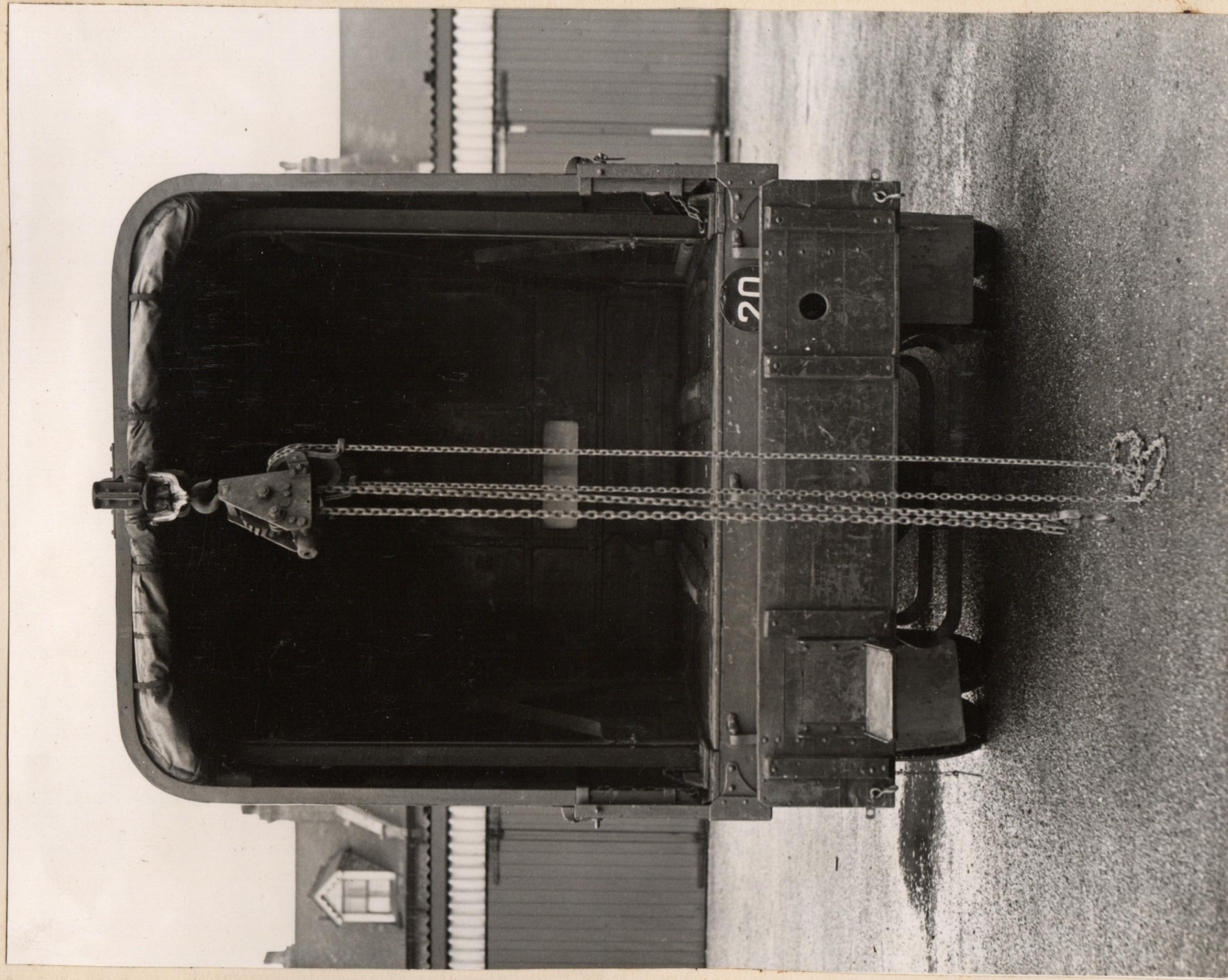
666B REAR VIEW SHEWING GANTRY & HOIST
