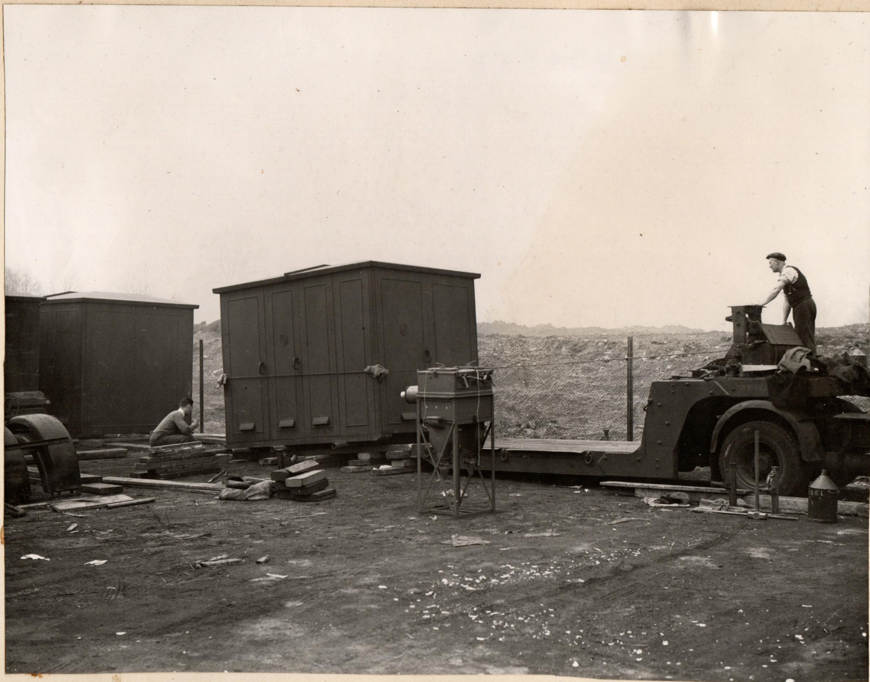
UNLOADING 5 TON ELECTRICAL KIOSK FROM 603 P - ALDENHAM WORKS
