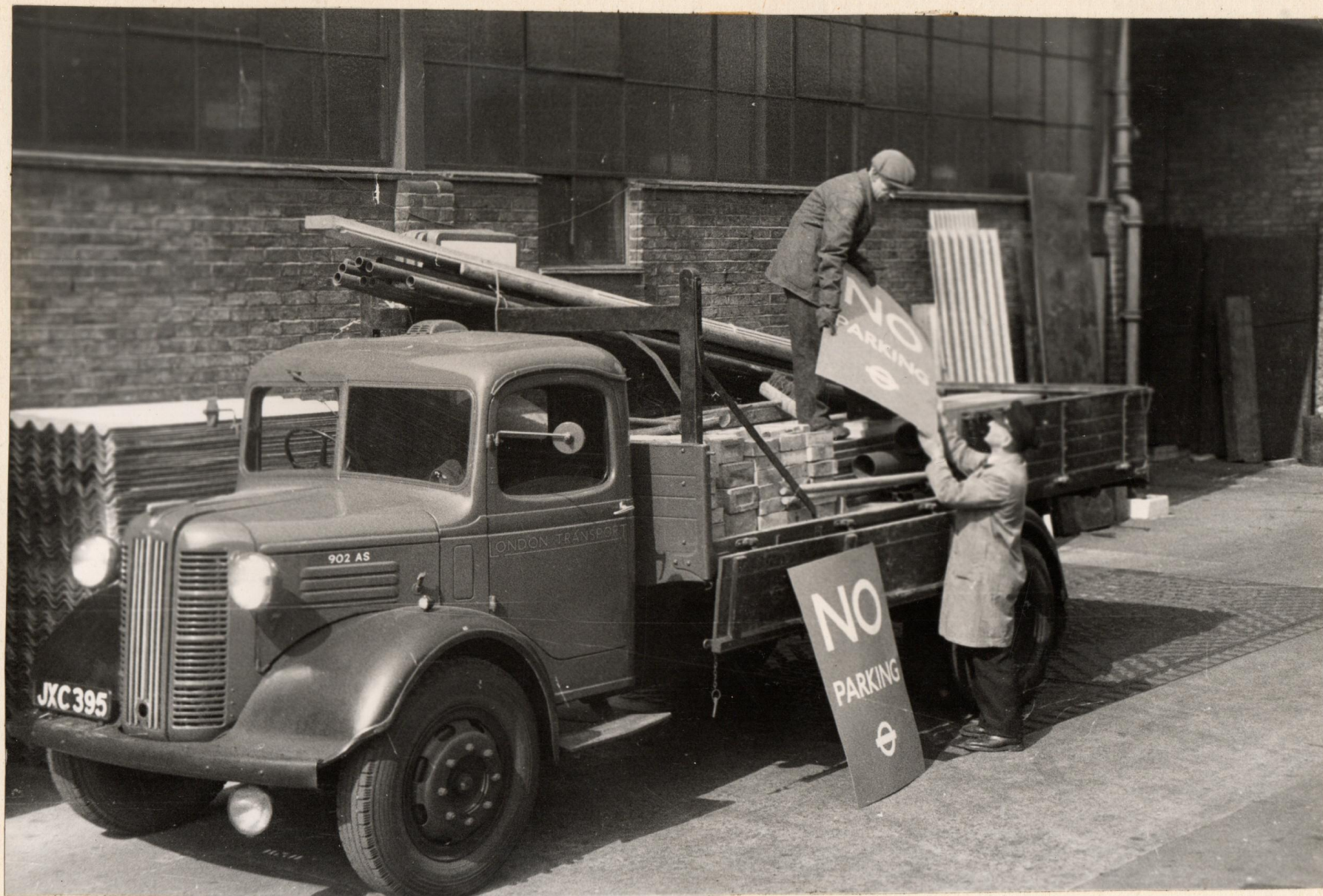
LOADING GENERAL BUILDING MATERIAL- PARSONS GREEN DEPOT
