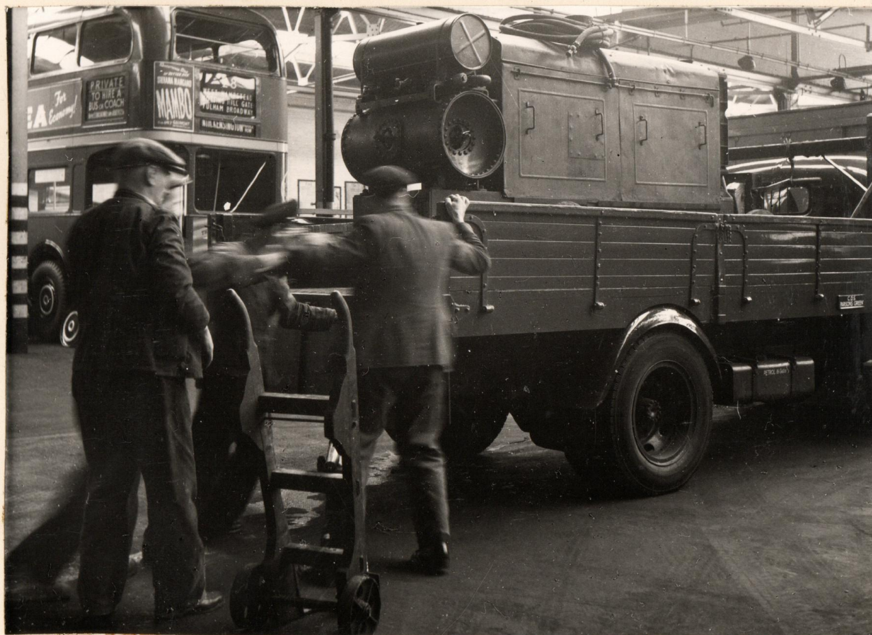
COMPRESSOR ON LORRY
