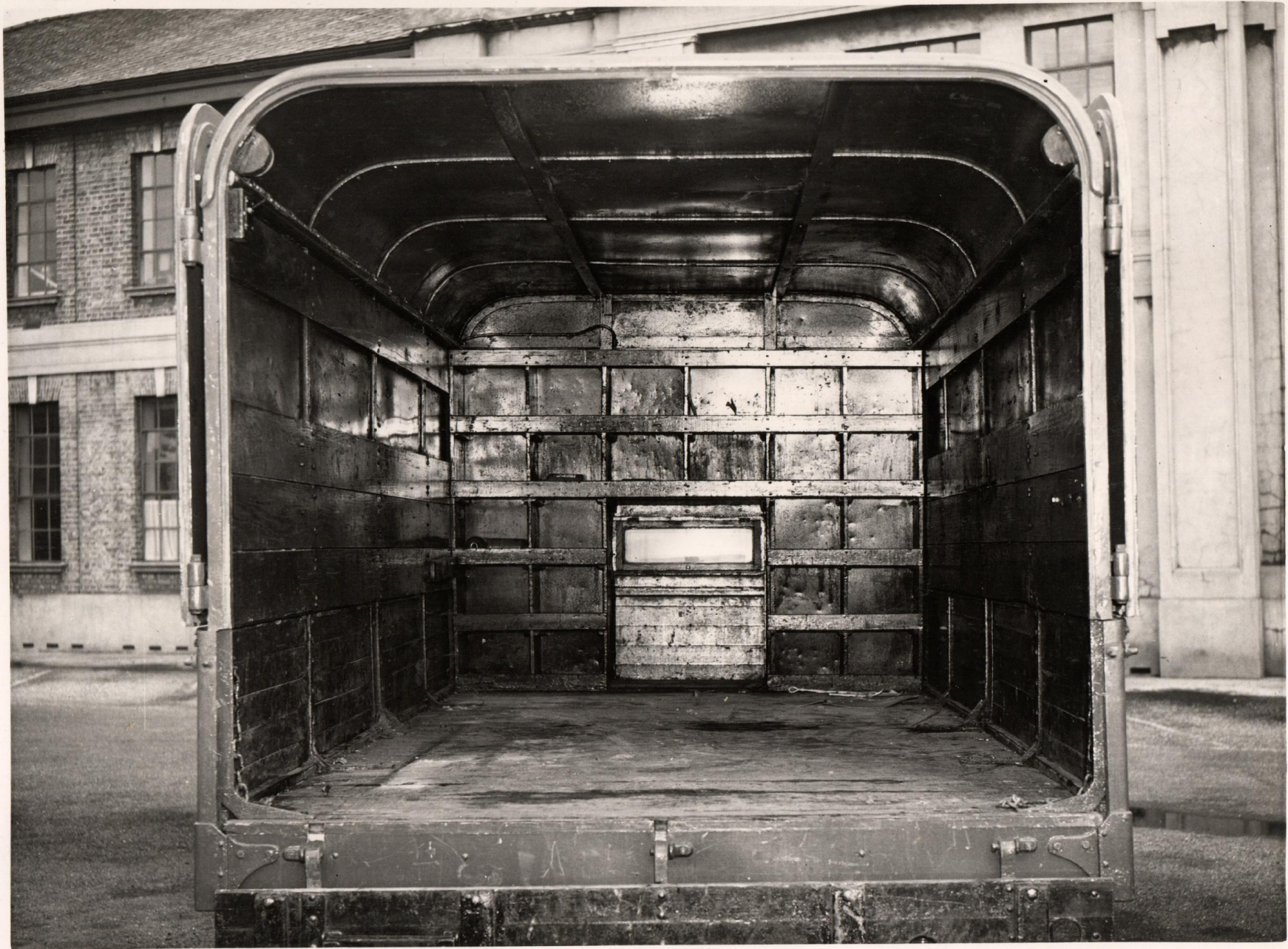
EX. PERMANENT WAY TRAM 5 TON BEDFORD FITTED WITH REAR DOORS
