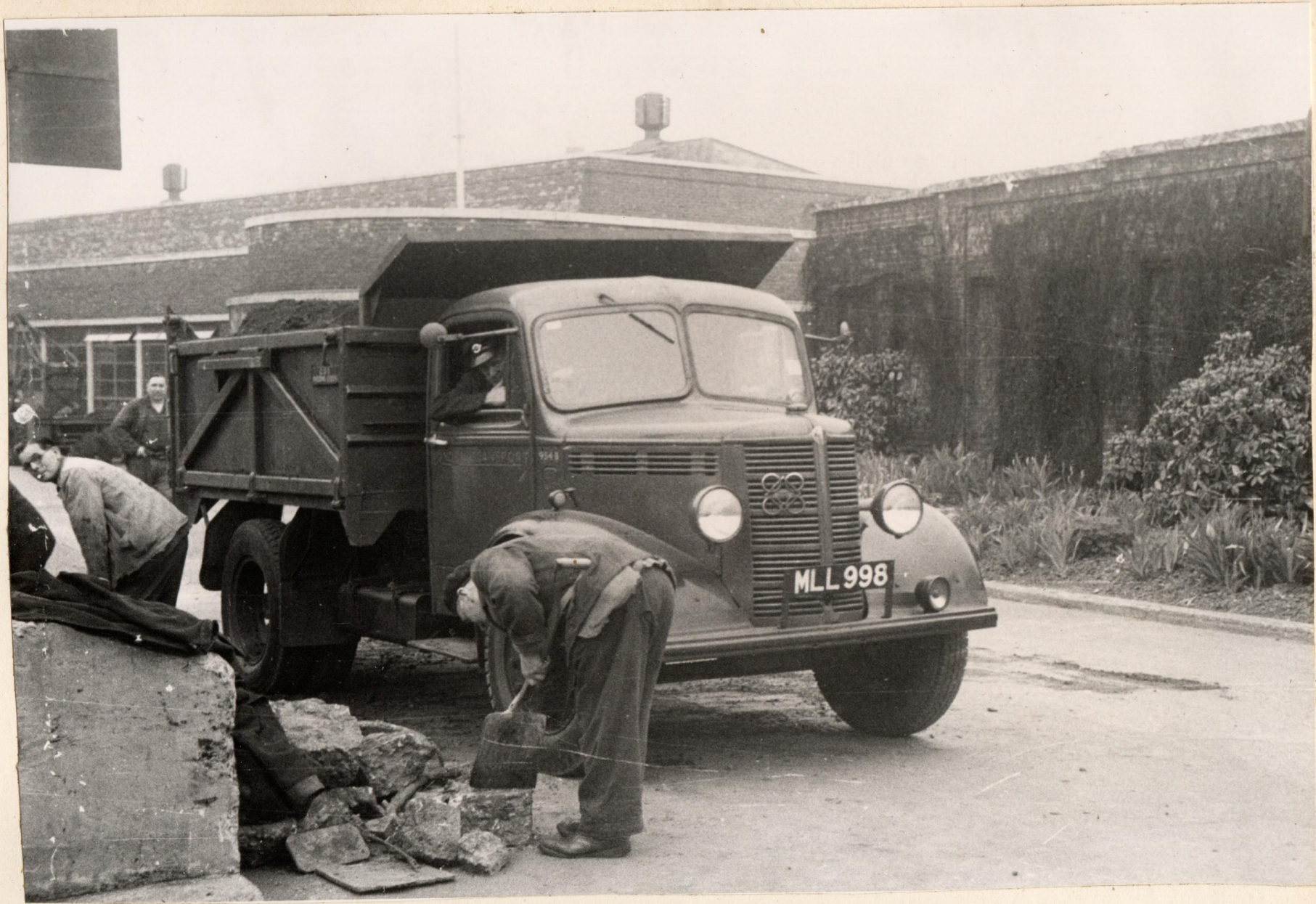
LOADING HARDCORE INTO CDS TIPPER - ACTON WORKS
