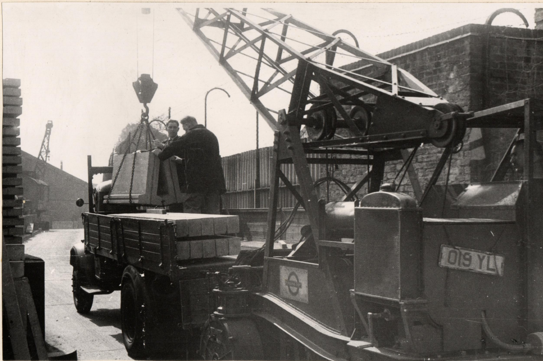
CDS 5 TON BEDFORD LORRY LOADING CONCRETE CASTING-PARSONS GREEN DEPOT
